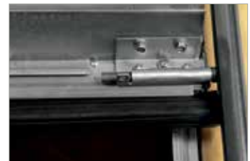
Bottom section roller slide attached to U-bar resists inward and outward force.
